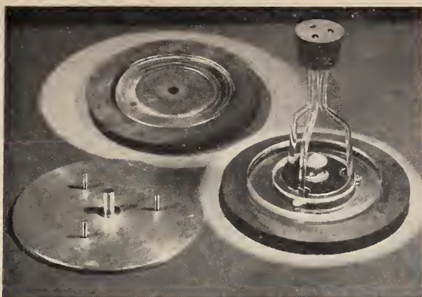
FIGURE 8. Bakelite holders for resist-coated circles.
