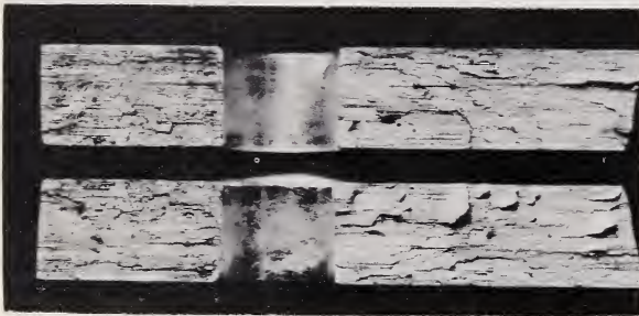
FIGURE 35.2. Portion of one of the cracks shown in figure 35.1 opened to show the fracture surfaces.
