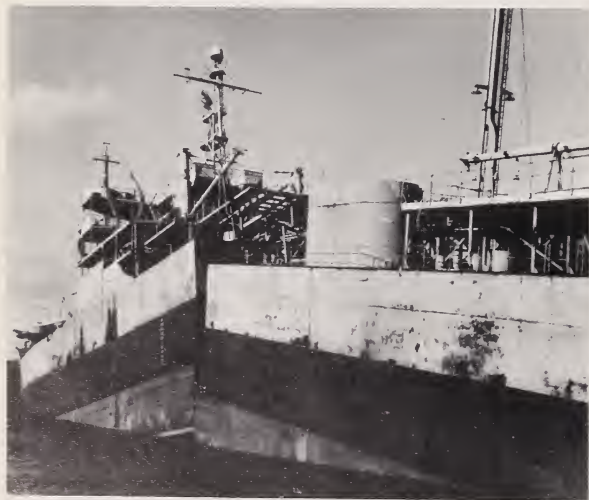
FIGURE 14.1. Tanker that broke in two at dock, viewed from port side.
