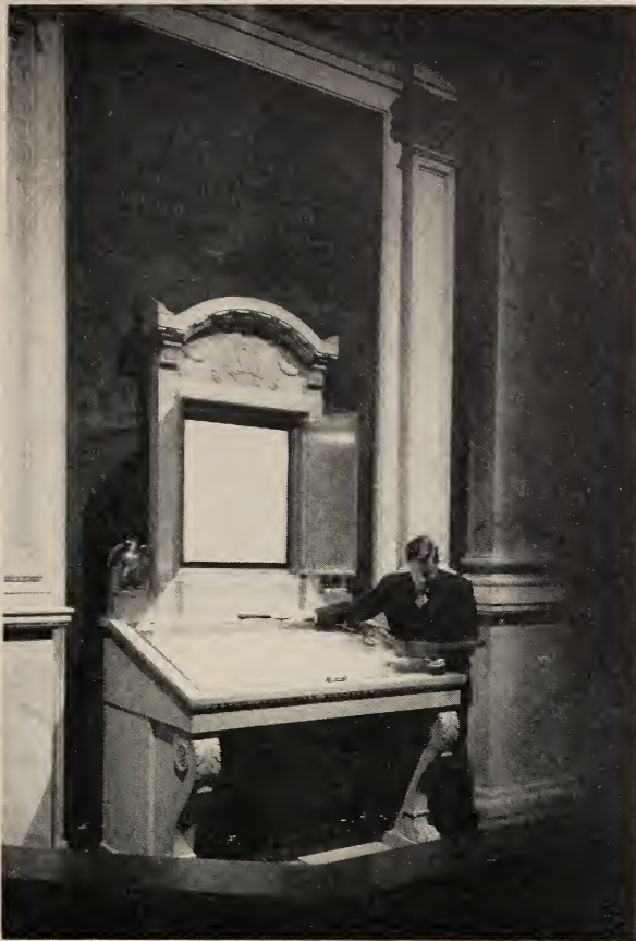
Figure 2. Adjusting the lights for an illumination of 10 footcandles by means of a photoelectric foot-candle meter.
