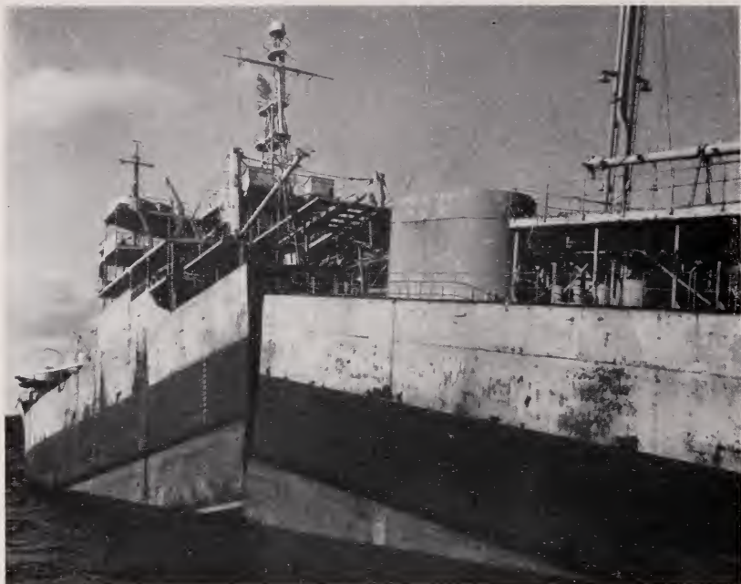
FIGURE 9.5 Tanker that broke in two at dock.
