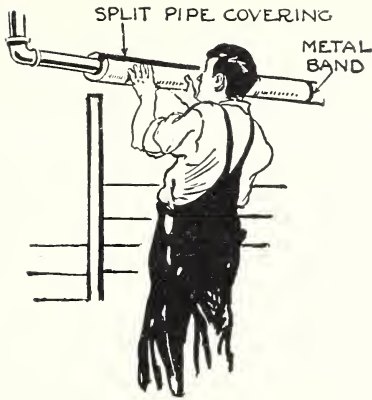
FIGURE 37.—Applying split pipe covering around hot-water heating pipes.
