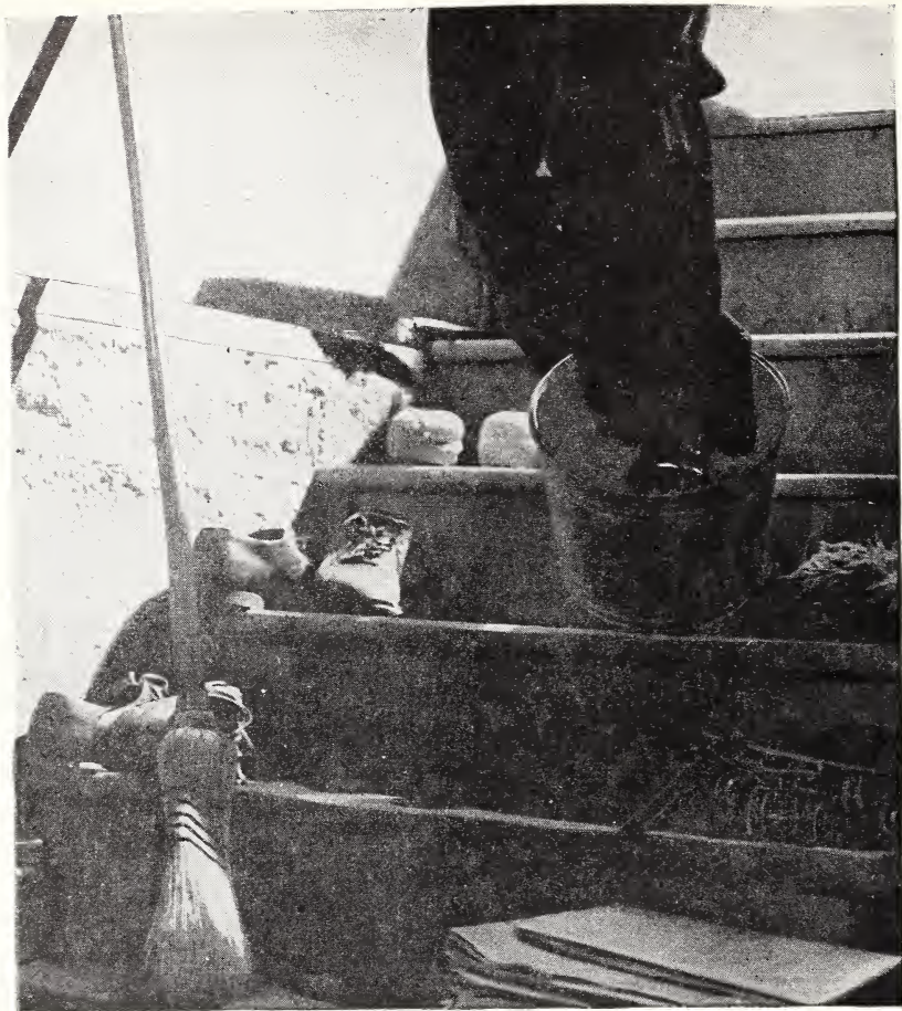
FIGURE 3.— Stairways such as this are decided hazards.
