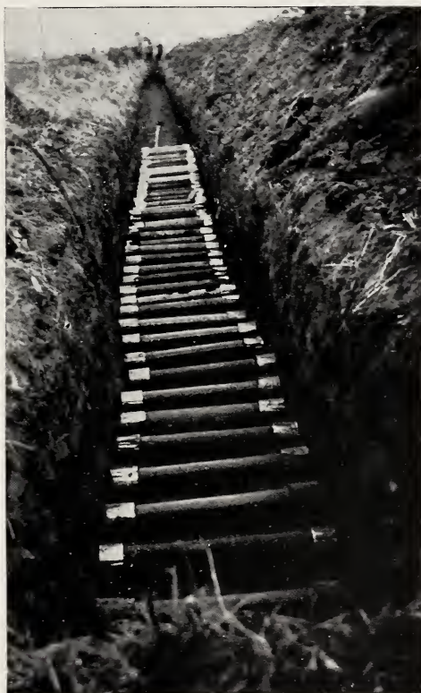
FIGURE 38.—American Gas Association coatings before burial.
