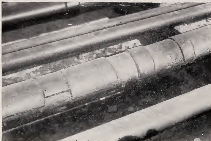
FIGURE 21.—“Half-sole” (welded patch) method of pipe repair.
