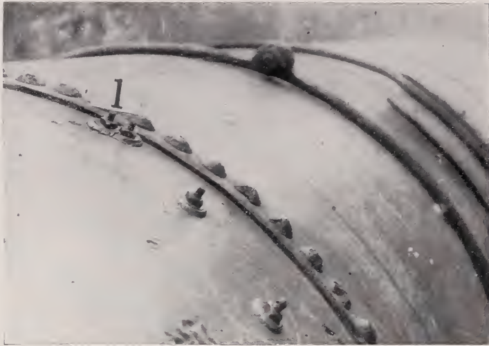
FIGURE 19.— Three types of repairs on a water line.
