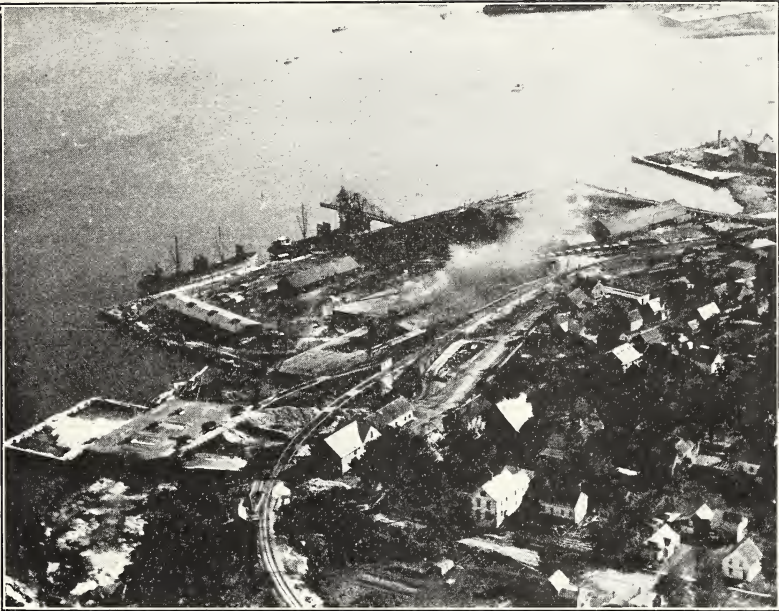
FIG. 20.— Plant and docks of the Rockland & Rockport Lime Co., Rockland, Me.
