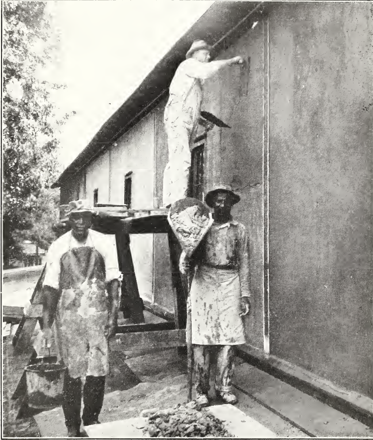
FIG. 7.—Applying the finish coat to a stucco test panel
