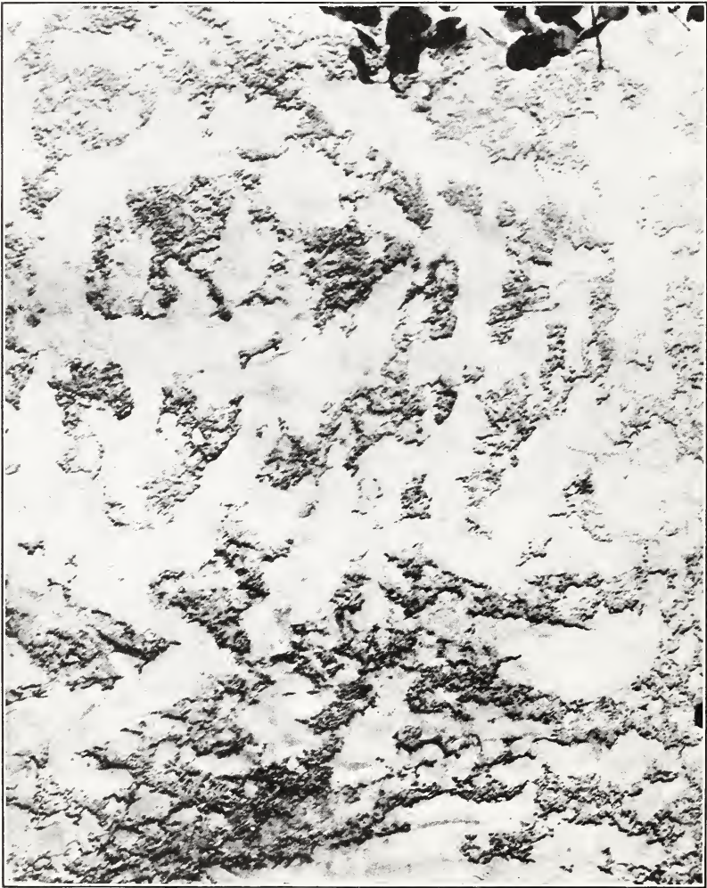
FIG. 13.— Floated rough-cast finish
