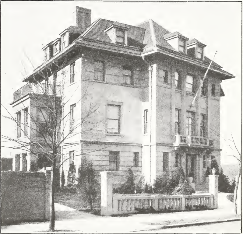
FIG. 1.— An overcoat job on brick finished with exposed aggregate (Siamese Legation, Washington, D. C.) (See fig. 14.)
