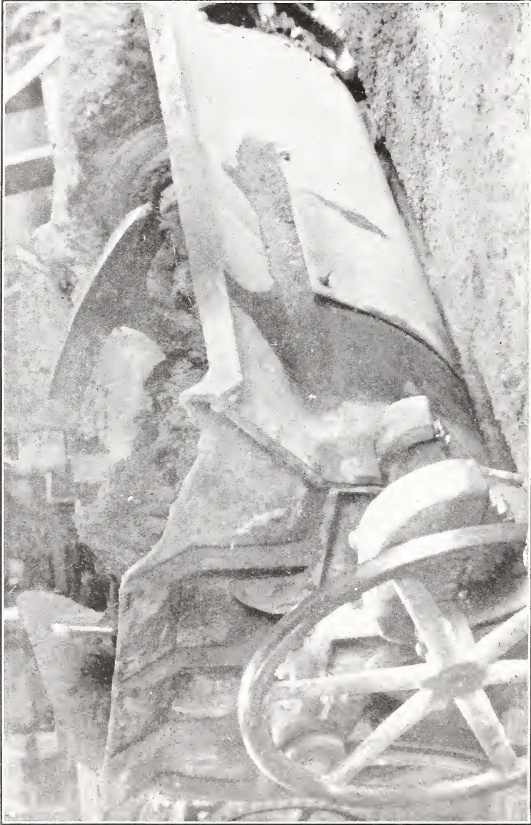
FIG. 4.—A charged concrete mixer of the revolving-blade type which is particularly well adapted for mixing dry concretes and mortars
