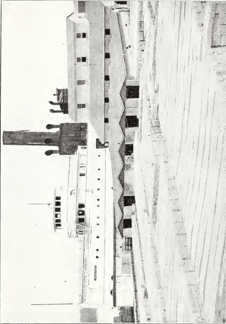
FIG. 8.—A well-designed concrete products plant showing the location of the six steam curing chambers between the plant proper and the storage yard
