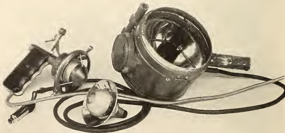
FIG. 14.— Electric lamps for daylight transmission of messages
