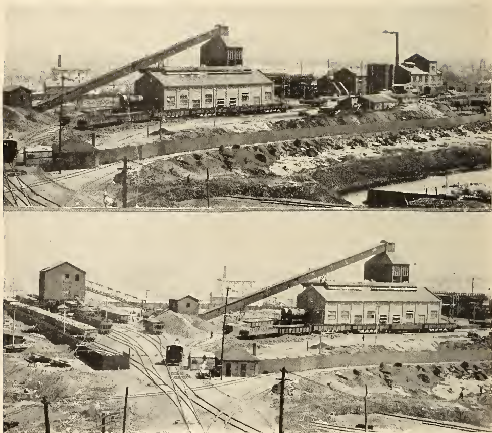
FIG. 8.— Two views of the Dover By-Product Coke Co.'s plant at Canal Dover, Ohio
